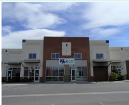
small-scale industrial/ warehousing
